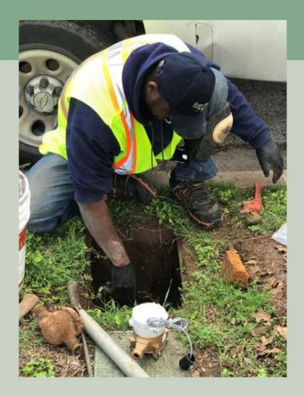
Replacing an inline water meter, a water meter setter, or gooseneck, pigtail, or connector
