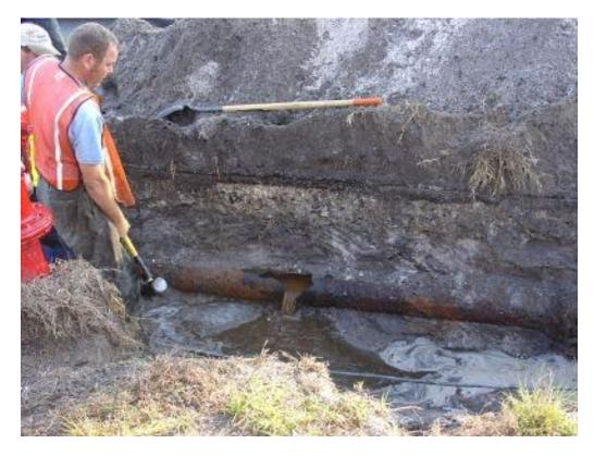
~8 AM: the main is decommissioned Equipment set in-place - rods paid out through the host pipe
