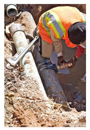
New services lines installed using a piercing tool
